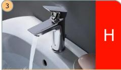
TAPS: Run individual taps for 6 minutes weekly- run cold for 3 mins & run hot for
