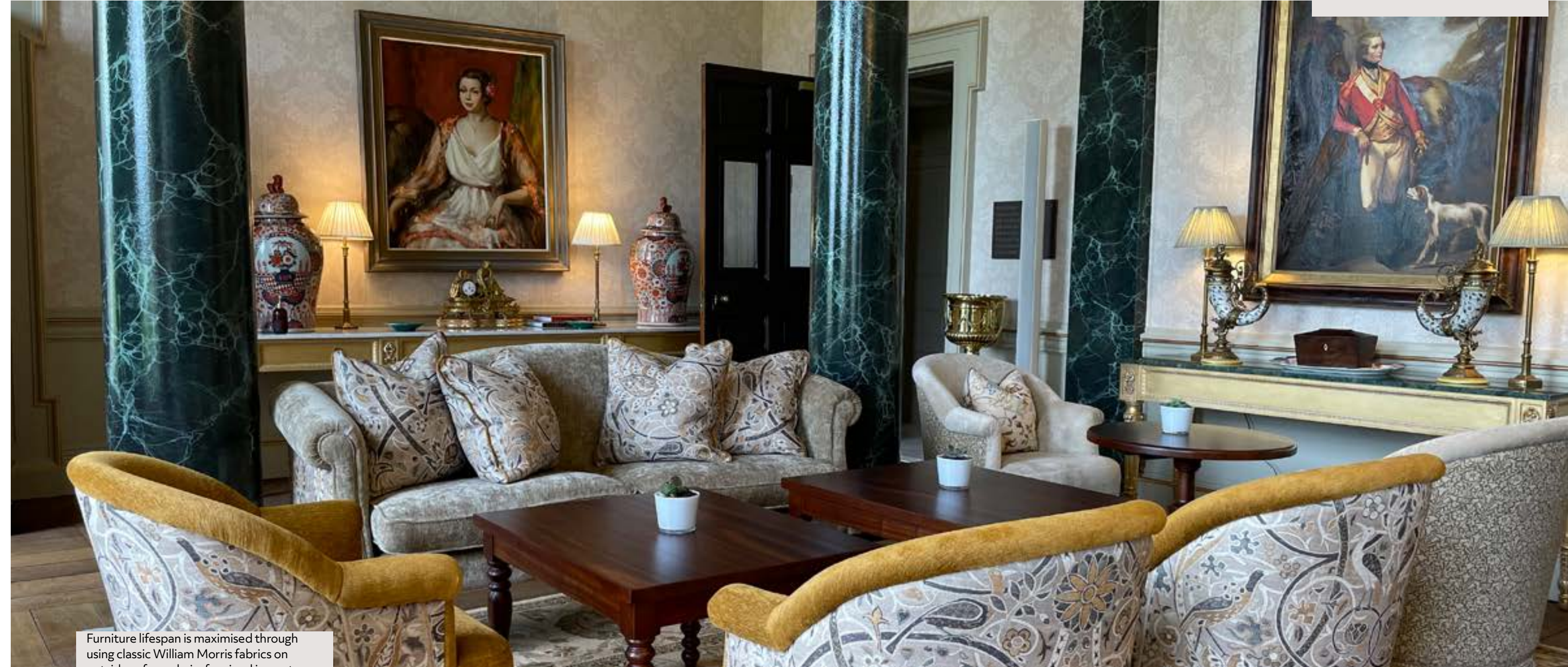
Specialist decorative painters were brought in to simulate marble surfaces in lieu of expensive natural stone.
