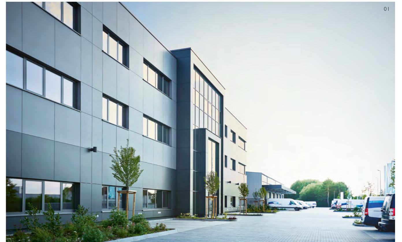
01 The new administrative and logistics building 02 Our reception area in Ille style
